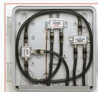
Typical VoIP or Cable Modem Installation
