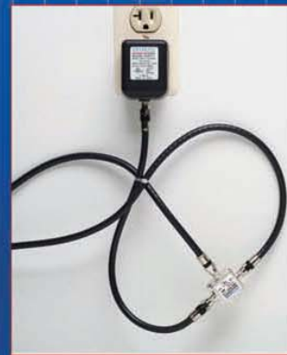
Typical Power Inserter Installation
